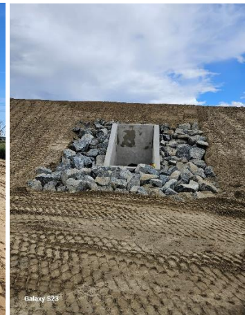
B Ditch Extension
